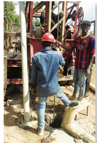
Top: A newly drilled well with protective wall; Bottom: Kobonal Water Project
